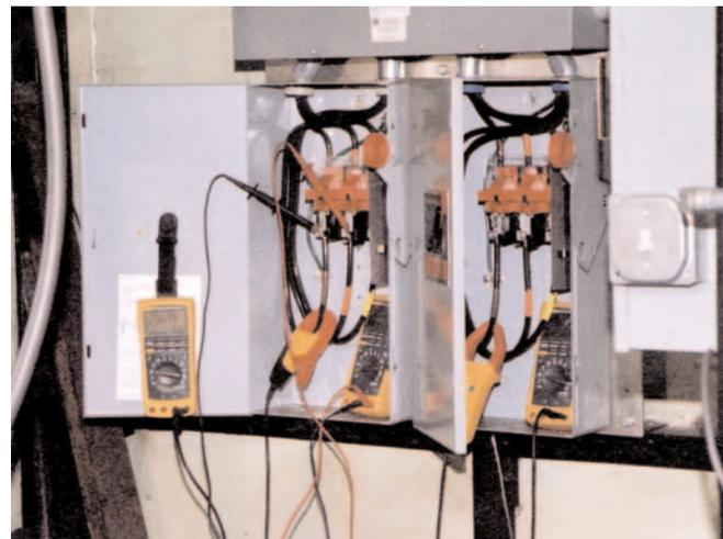
Simultaneous current and voltage logging at the control panel for two drive motors.
